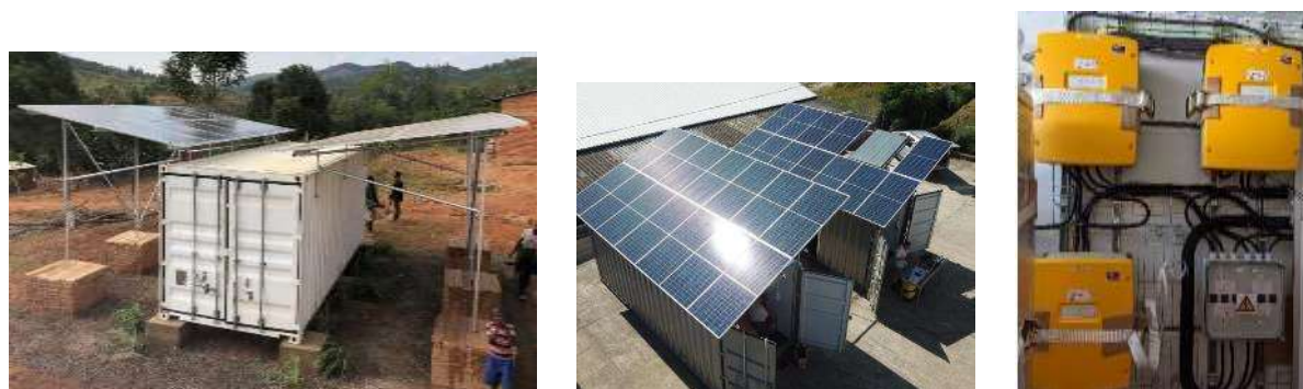
Figure 75: From left to right: Examples of two types of containerised off-grid solar systems, hybrid inverter
