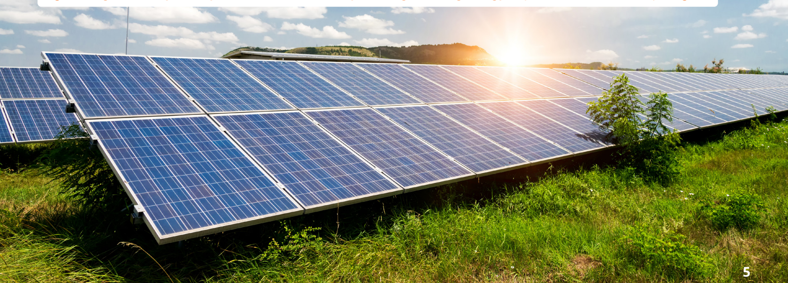
Figure 2: Agrivoltaic systems provide shade to the crops while generating energy (Diyana Dimitrova via Getty Images)
