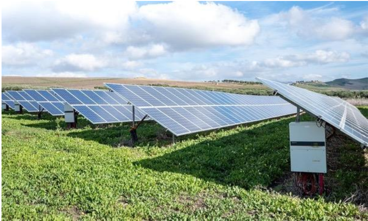
Figure 43. Agrivoltaic systems provide shade to the crops while generating energy (Adhiambo, 2022)
