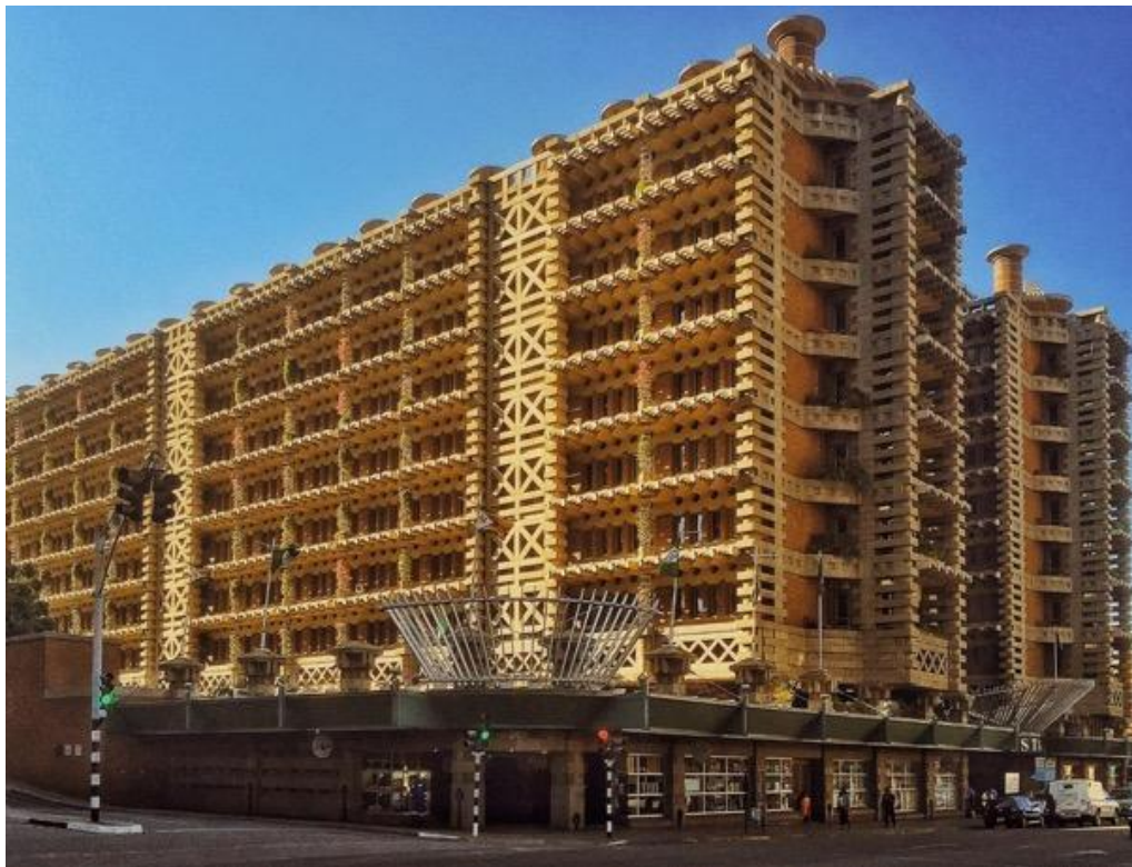
Figure 35. The Eastgate Centre, Harare, built in 1996 and one of the first large-scale buildings in the world designed to be ventilated and cooled by entirely natural means (Livin Spaces, 2018)
