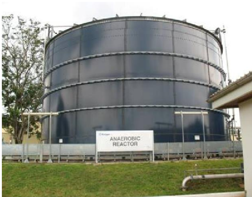
Figure 14: Biogas digester in Guinness Ghana Limited
