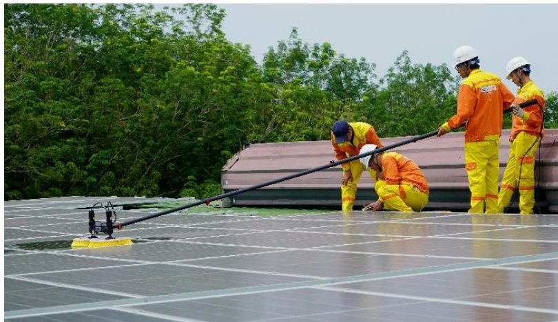
Figure 11: Solar PV maintenance. Photo by Trinh Trần on Pexels
