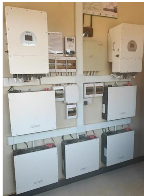
Figure 4: Actual solar system installation in health facility in Tanzania, photo by Elico Foundation.
