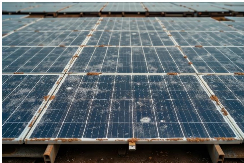
Figure 9: Dusty and Weathered Solar Panel Array © Vitalii Buria | Dreamstime.com
