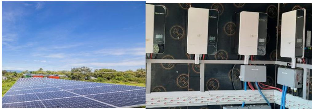
Aerial view of Kisegi ground mounted solar panels and hybrid inverter system
