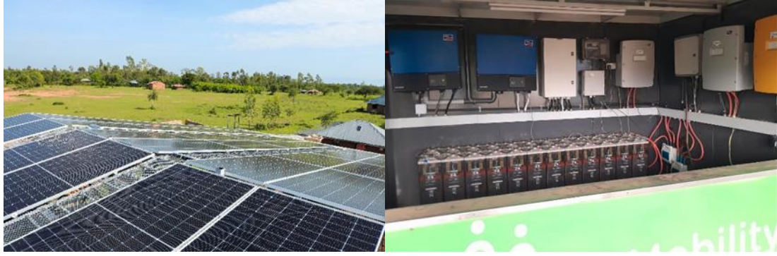
Aerial view of roof mounted Katito solar panels and traditional SMA inverter system
