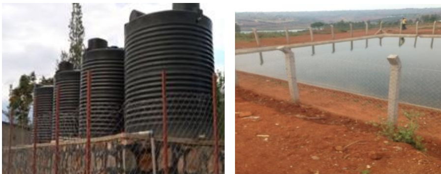
Figure 4a, 4b: Elevated and surface storage water tanks (source: Anonymous, field photos from Bugesera District, Rwanda).
