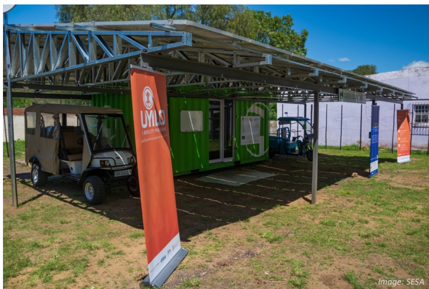
Figure 10. Off-grid solar containerised energy system with electric vehicles in Alicedale (South Africa)
